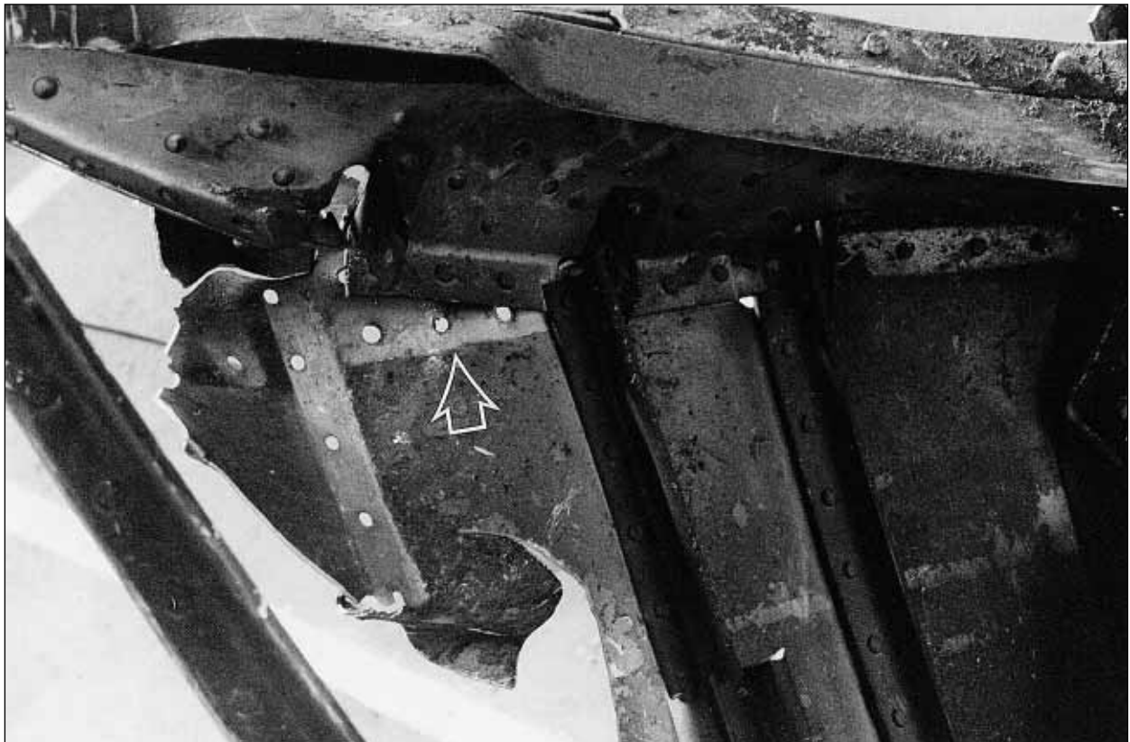
Figure 5. Exposed internal skin showing airborne fire sooting. Areas free of soot (arrow) indicate where overlapping metal was pulled apart at impact.
