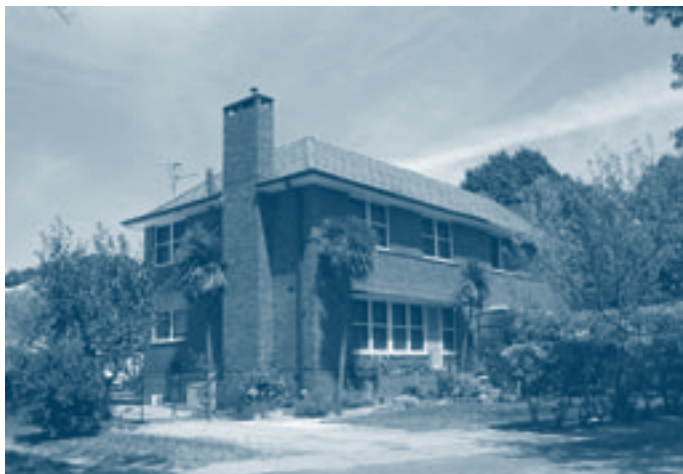
An original dwelling in Narrabundah (Photo: ACT Planning and Land Authority)
